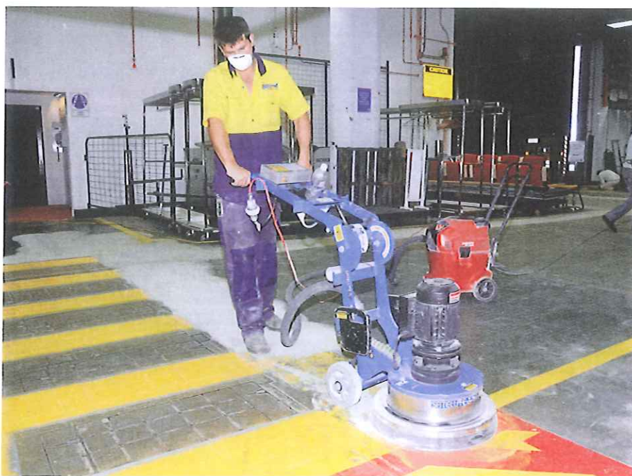
Scott Peatman removes layers of line markings dating back 40 years.
