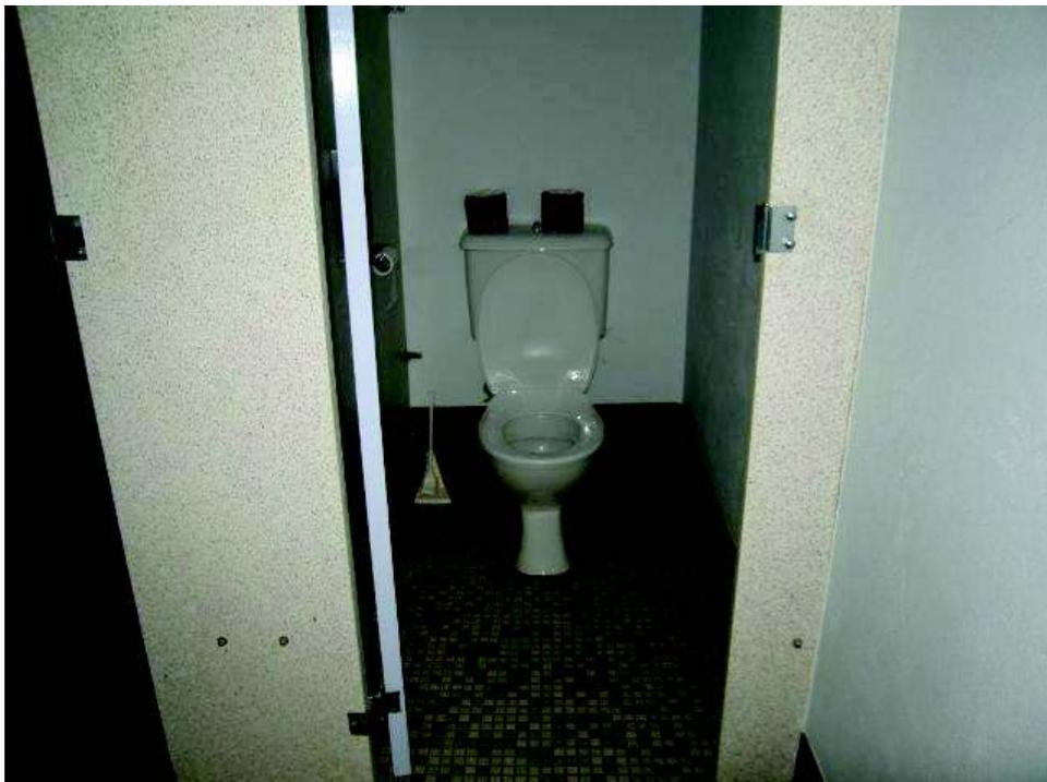
**Figure 12** Photograph of interior of office building – Toilets do not have dual flush cisterns and the floor and wall tiles require replacing.
