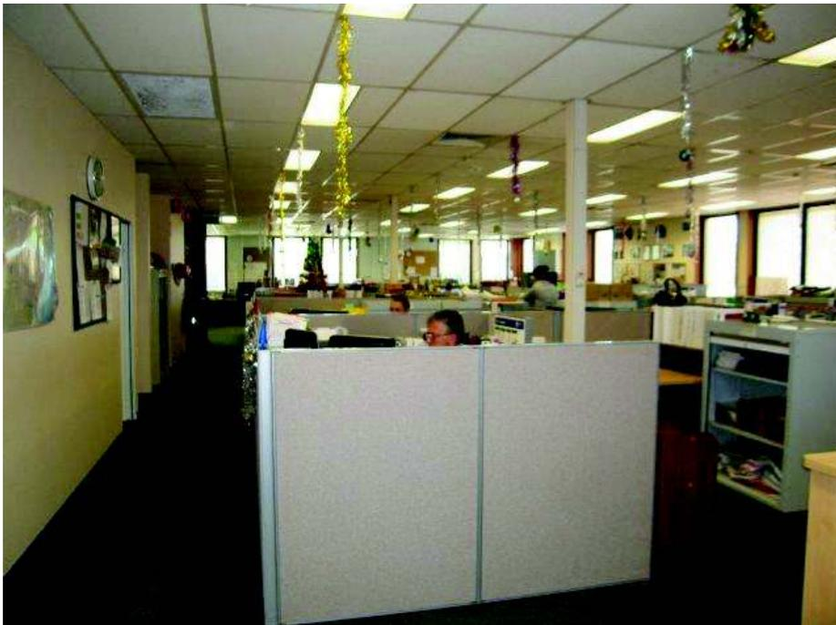
**Figure 10** Photograph of 4.002, (same condition as 4.003, 4.005 and 4.006) - Ceiling grid and tiles require replacement due to their condition and the water marks.
