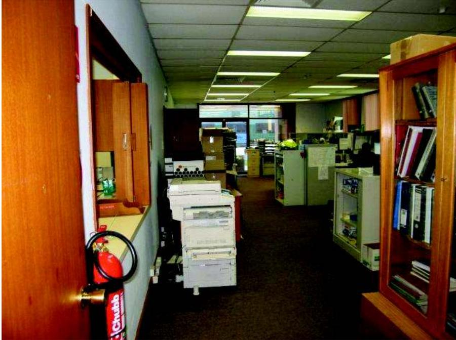
**Figure 7** Photograph 1.001, (same condition as 1.002, 1.003, 1.004 and 1.011) Ceiling grid and tiles require replacement due to their condition and the water marks.
