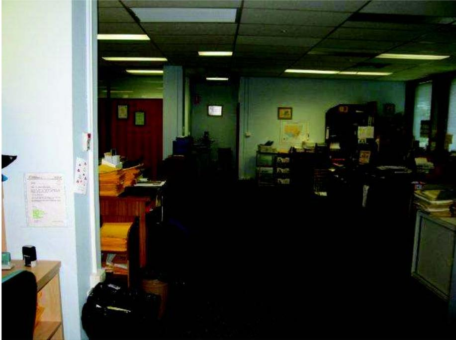
**Figure 9** Photograph of 3.003, (same condition as 3.001, 3.002, 3.004, 3.005, 3.008, 3.009, 3.010, 3.011, 3.012, 3.013, 3.014, 3.015 and 3.016) Ceiling grid and tiles require replacement due to their condition and the water marks.
